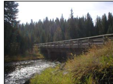
Photo 3.2 Grayling Creek Bridge Looking Northwest
