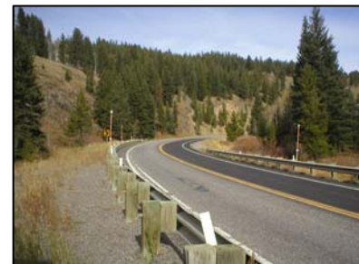
Photo 3.4 Road through the Proposed Project Area Showing Guardrails
