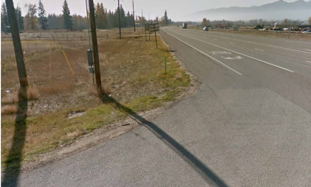
Figure 3. Looking South from Bell Crossing past the Stop Bar
