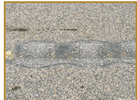
Example image of completed cut
